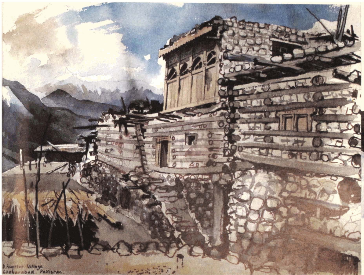
Left A house in Khurtlot village painted in water-colour (above) by Ian Davis. Note horizontal timbers giving lateral flexibility.
